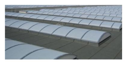
**POLISHIELD WHITE** contains pigments that reflect the sun's infrared heat, absorb ultraviolet light, but are translucent to visual light. It protects buildings from overheating by reflecting a large portion of direct solar energy, while maintaining high light transmission.
